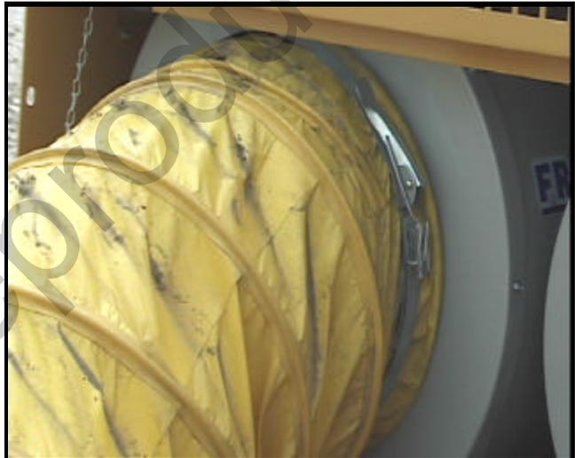
16" over-center band clamp (pn848174) used here to attach duct (pn848172)
